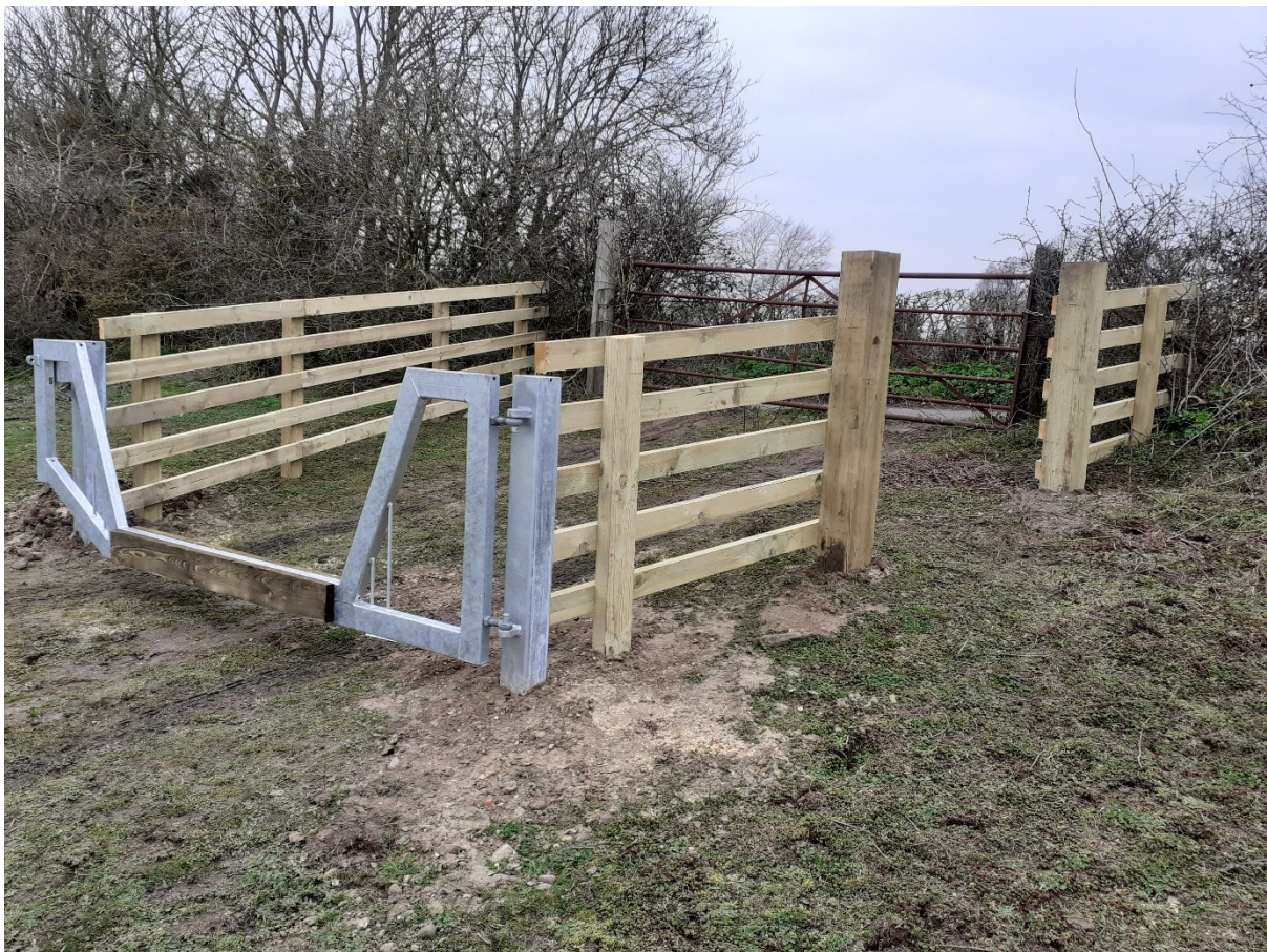
Hall Lane vehicle access and 'horse stepover' gate ( Kissing gate to be added )
